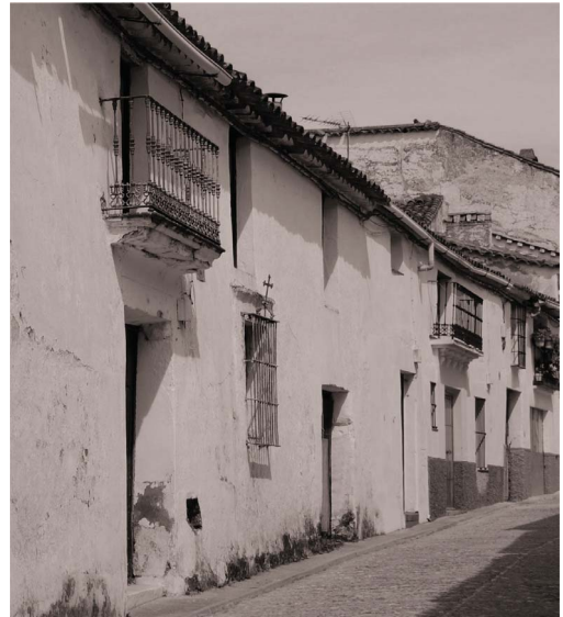
Figure 3. Limed wash façade on andalusian popular architecture. Aracena, Huelva (Rodríguez García, 2011).
