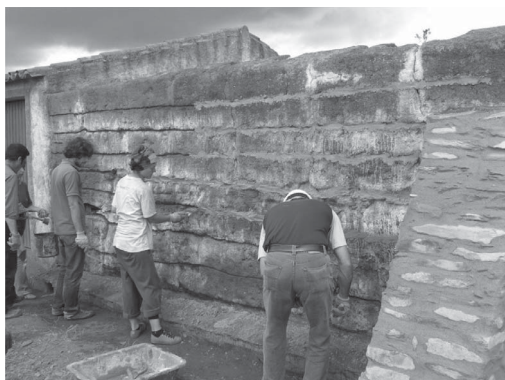
Figure 5. Course of bio-construction: earth plaster workshop (Canivell, 2006).
